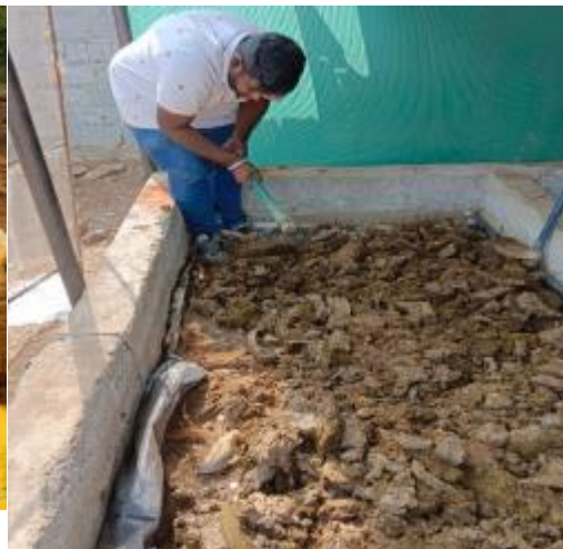
BASE PREPARATION FOR PIT
